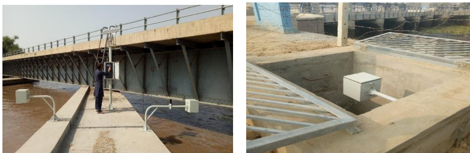
Figure 4: RTFM Sensors installed at Eastern Sadiqia & Fordwah Head at Suleimanki Barrage and at Jalwala Head
